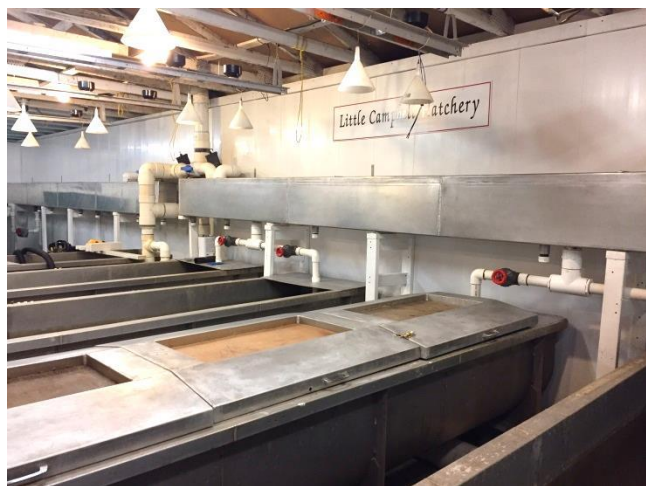
New head troughs and wall paneling
