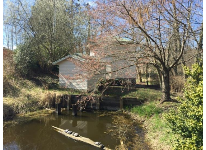
Water tower in the background with the well/pump house in the foreground.
