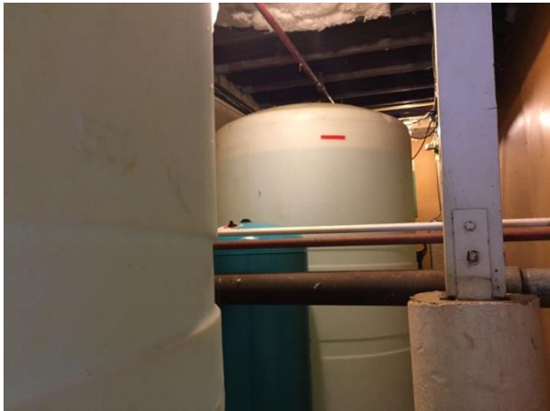
A view of the secure 500-gallon reverse osmosis filtration system.
